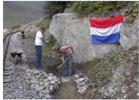
Picture 1: Dutch voluntary workers creating drainpipes.
